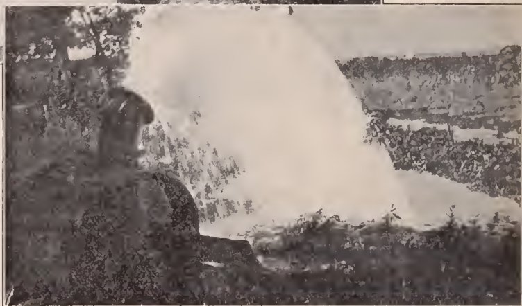
Irrigating well. Irion County, Texas, ca- pacity 4,000 gallons per minute.
